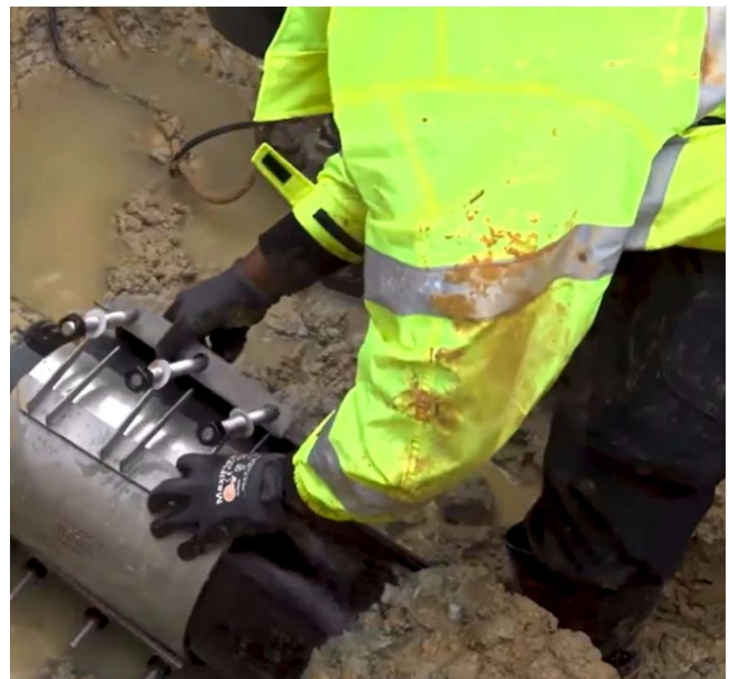
Repairing a water main
